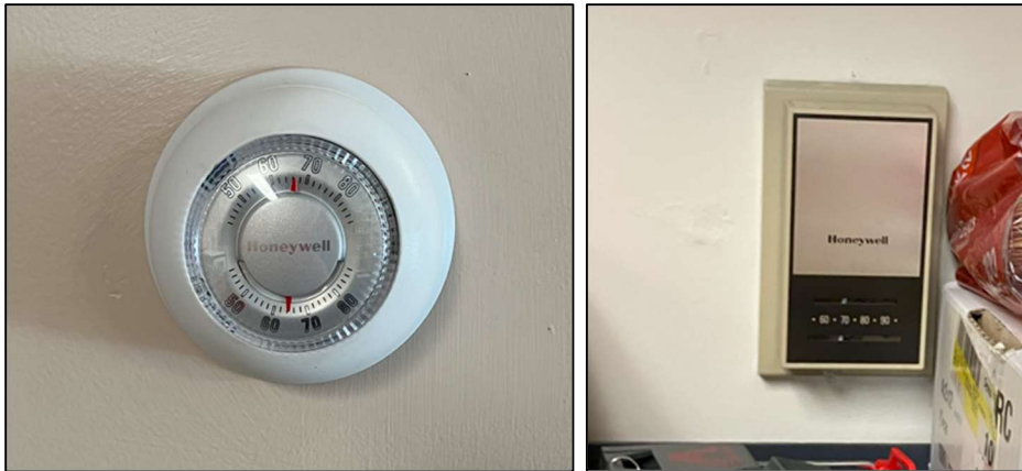
Existing thermostats in office and food pantry
